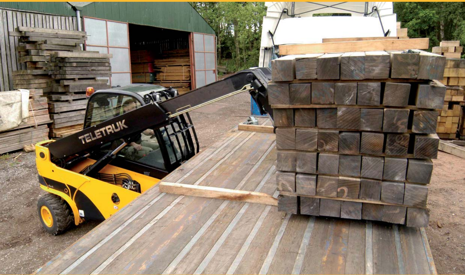
4x4 Teletruk reaching forwards, loading the lorry from one side only
